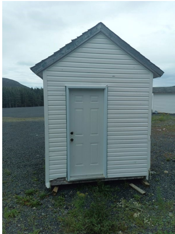
Picture 1 - Front View
